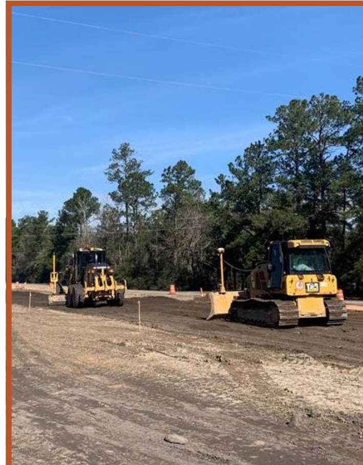
The contractor grades limerock in preparation for paving.
