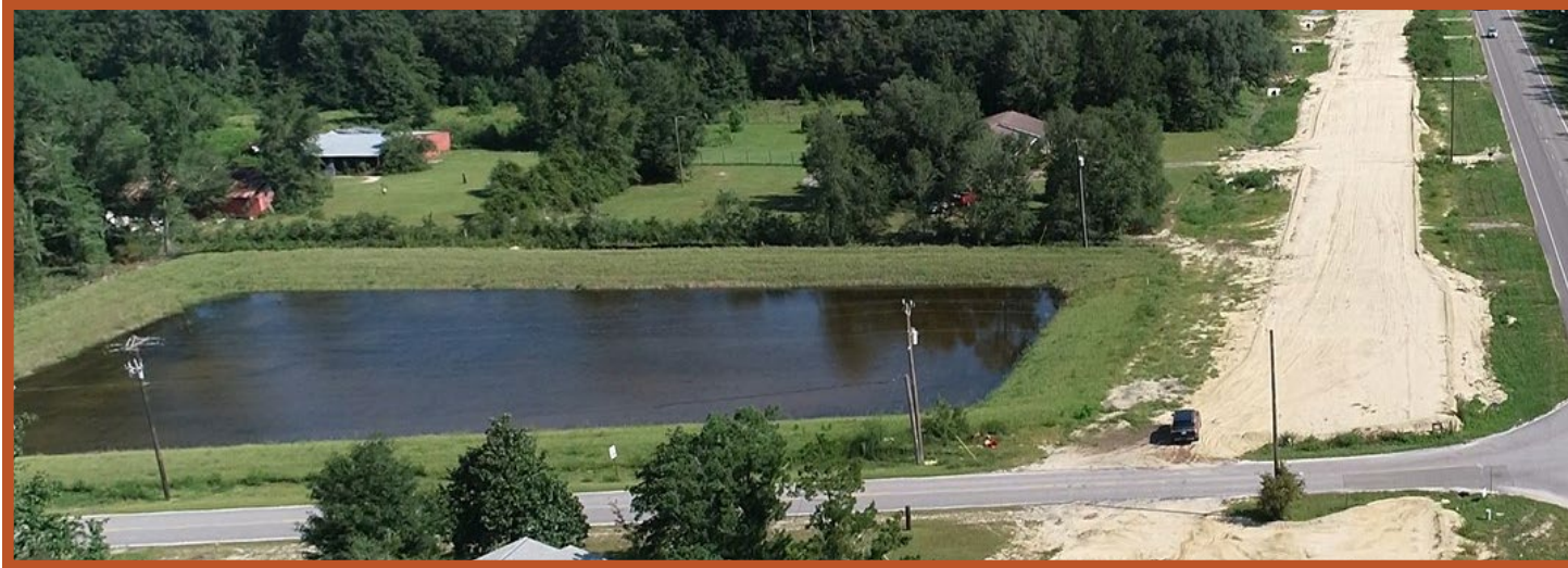
Stormwater pond near Chain Lake Road.
