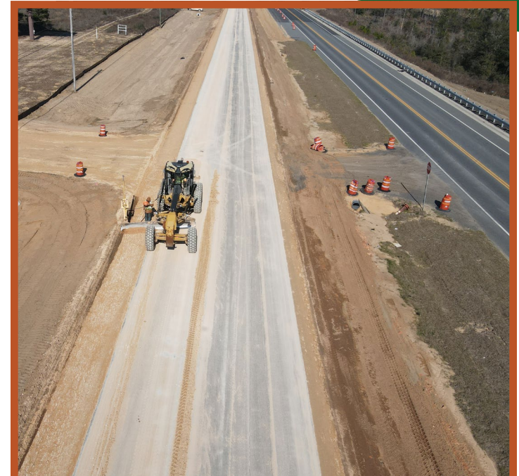
The contractor grades limerock in preparation for paving.
