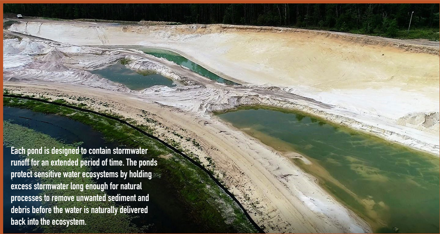
Westbound aerial view of the stormwater pond near the Chain Lake Road and S.R. 77 intersection.
