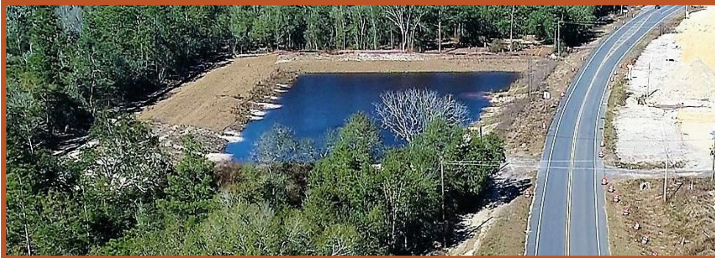
Aerial view of the stormwater pond located just south of Moss Hill Road.
