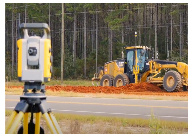
(TOP and MIDDLE) The arrows in these photos point to the motor grader's GPS technology used to control the roadway's grade during construction. The system measures the height of the material to ensure the material spreads evenly.
