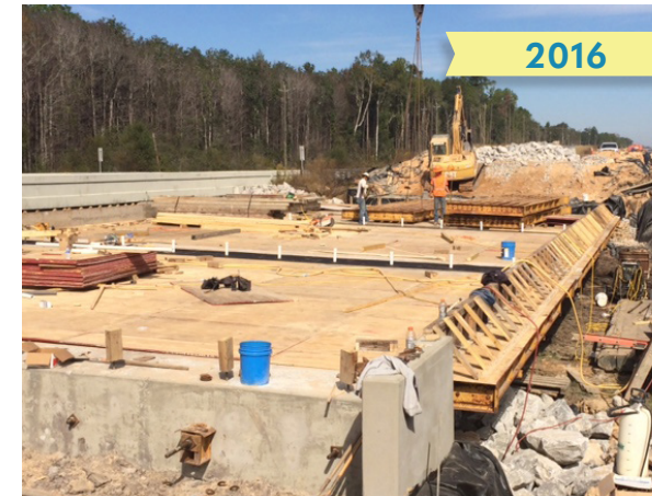
(LEFT) Open Creek Bridge under construction in 2016.
