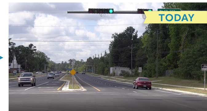
(LEFT and RIGHT) Part of the S.R. 79 at S.R. 277/Court Avenue intersection upgrades include removal of a raised median.
