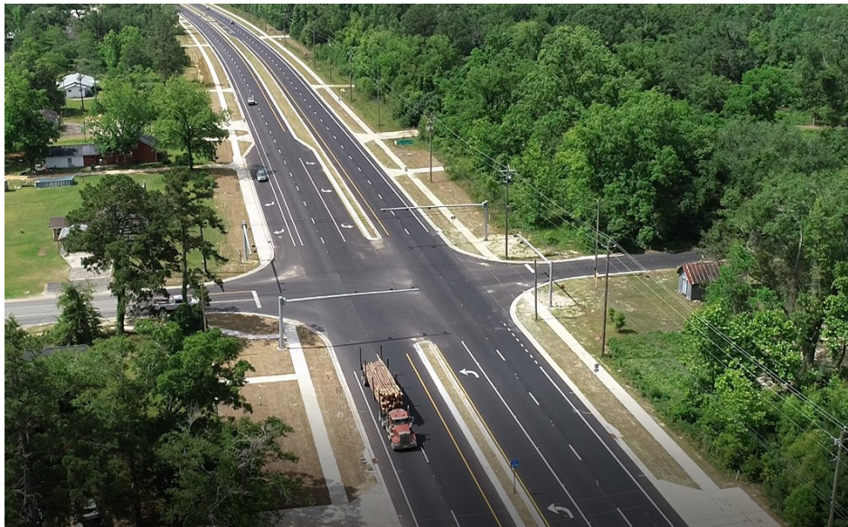
(ABOVE) C.R. 279/Moss Hill Road intersection today.
