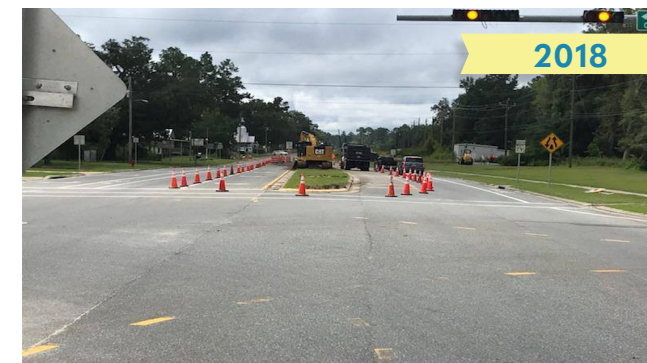
(LEFT and RIGHT) Part of the S.R. 79 at S.R. 277/Court Avenue intersection upgrades include removal of a raised median.
