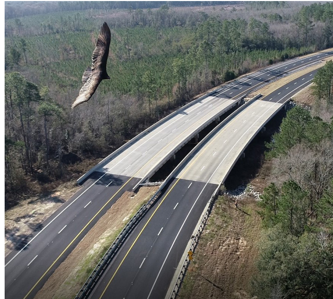
(ABOVE) Aerial drone technology captures a bird of prey flying over Cypress Creek Bridge.
