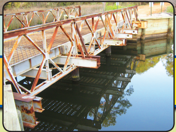
Existing Turkey Creek Bridge
